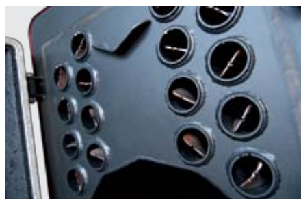
Ash extractor: tubes
