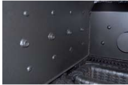
Post combustion air inlet holes
